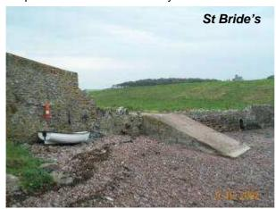
sections of very local defence, patching up where sections of the low cliff and bank have eroded. There is a steep slipway associated with the main wall. They are in moderate to poor condition and are being undermined with only some areas fronted by a natural beach. In other areas of the zone there are minor works associated with the ferry landing stages on Skokholm, Skomer and St Martins Haven.
