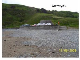
The bay is well sheltered from the west but is exposed to waves from a north westerly direction. Beach levels can vary and the wall does have a significant local effect in tending to direct wave action into the valley and also along the face of the wall to the north. In effect the eastern end of the wall acts as a small smooth headland dividing and redirecting wave action. With sea level rise, the beach would attempt to roll back and will steepen against the sea wall. There would also be
