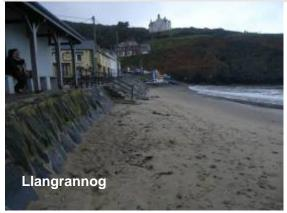
The main defence is a large stone masonry wall along much of the seafront, with the seafront road and properties immediately behind. The stream to the west is in open culvert and the main stream runs in open culvert beside the car park and flows through a closed culvert through the sea wall. The northern section of the bay is generally protected by a higher shingle bank with local private defences to property behind. The main sea wall is in moderate to poor condition, with the toe of the wall
