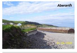
Located about 2km north of Aberaeron is the small rural village of Aberarth, situated on the same boulder clay platform as Aberaeron. It sits within the valley of the Afon Arth and the mouth of the Arth is artificially controlled by a crib groyne. A sewage pumping station for the village is situated on behind the crib groyne on the landward side of the steam behind a sea
