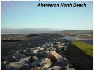
rock groyne and sea walls. These defences were constructed to prevent erosion of the north side of the harbour and to protect the town from coastal flooding by means of overtopping during storms. Along the shore where the groynes are in place, there lies a car park and a number of properties, together with the sewage pumping station and pumping main situated on a landfill site, which is now closed. It is anticipated that the groynes will stabilise the beach in front of the town
