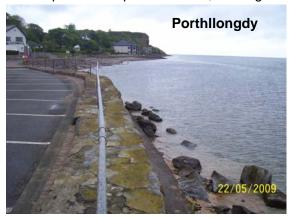
at Porthllongdy being indicative of the limit of significant way action. Locally, the various defences along this frontage may result in some scour and there is some overtopping, but overall the main processes will be the general distribution of sediments by interaction of the narrow channel and the massive intertidal sand banks.
