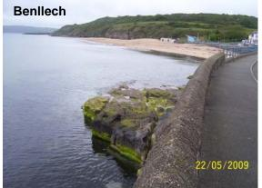
The southern end of the wall, despite the small areas of rock, is similarly exposed to the main wave attack and would tend to deflect waves into the beach area to the south. This wall is seen as having a significant local influence of the area.
